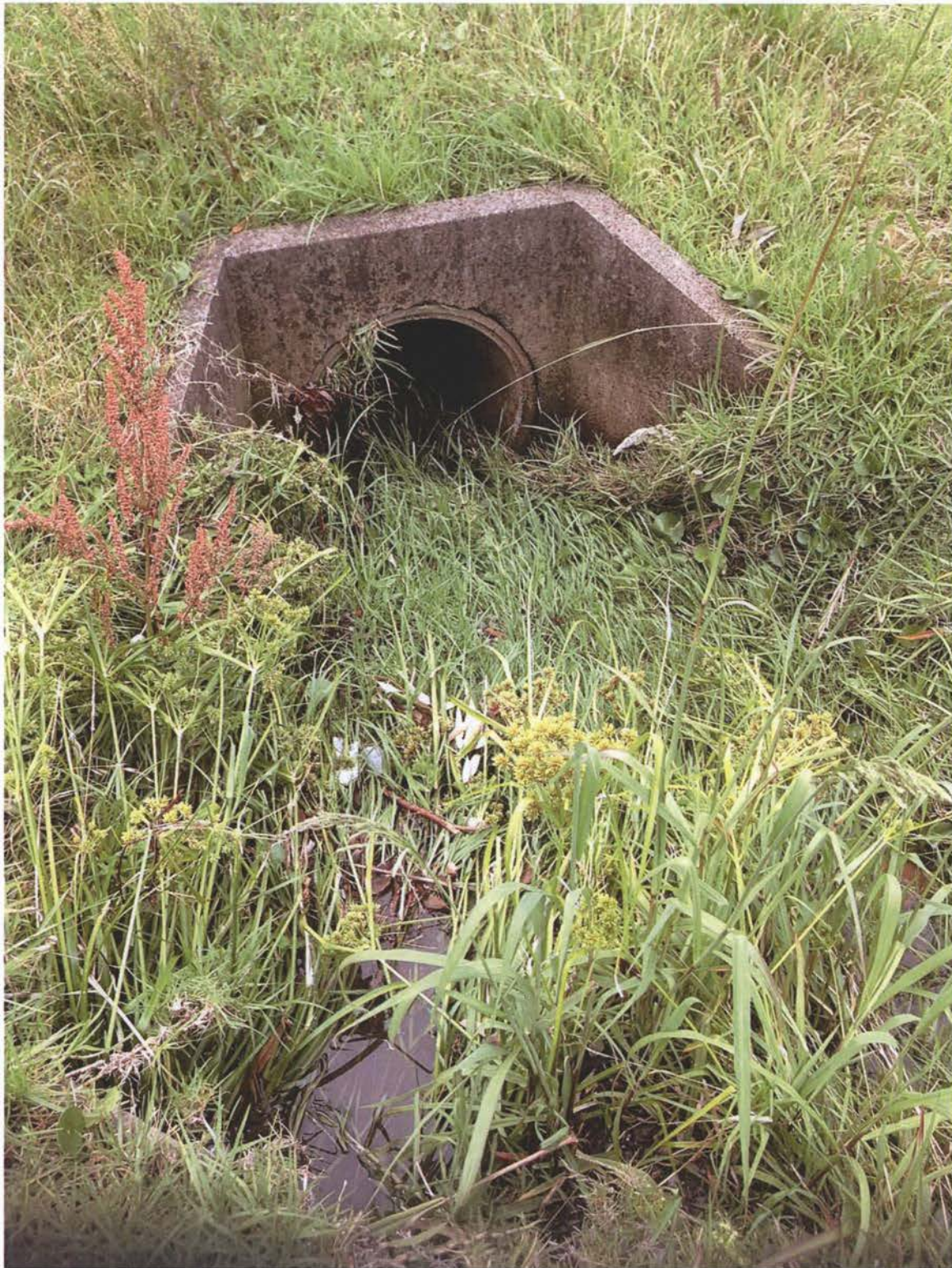
Photo 5 – Drainage line 1 – upstream stormwater culvert, commencement of watercourse
