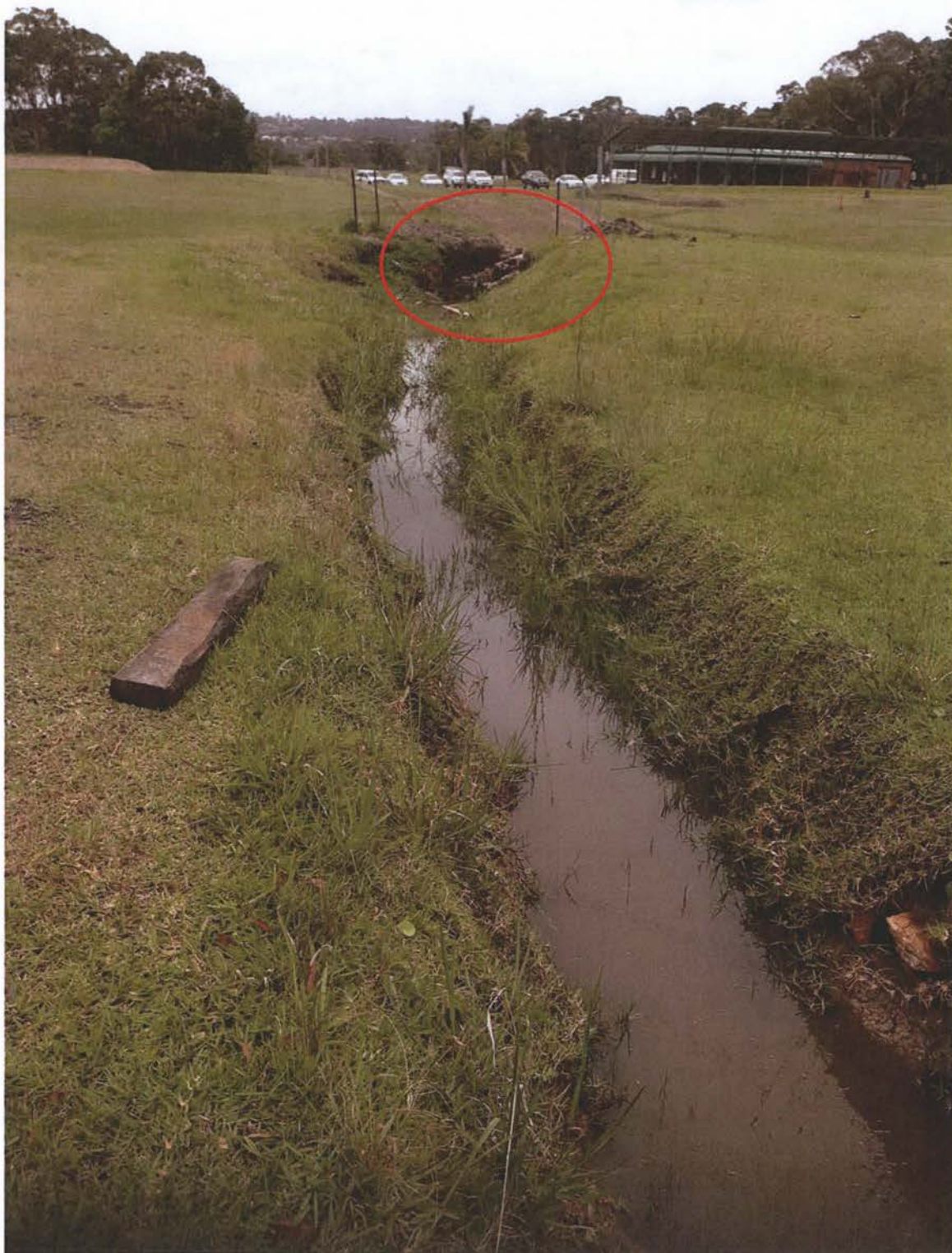
Photo 6 – Drainage line 1 – blowout at crossing
