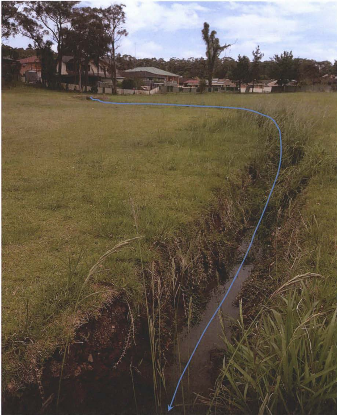
Photo 4 – Drainage line 1 - southern portion showing channelised portion with active bed lowering
