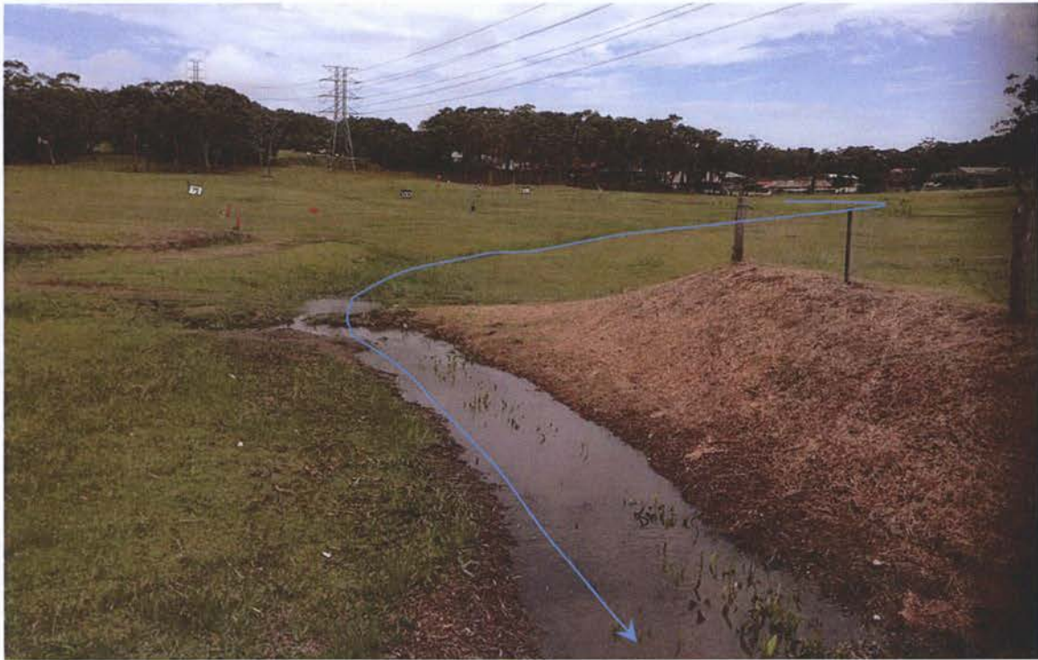
Photo 2 – Drainage line 1 - downstream portion showing fill on RHS but a stabilised natural formation channel
